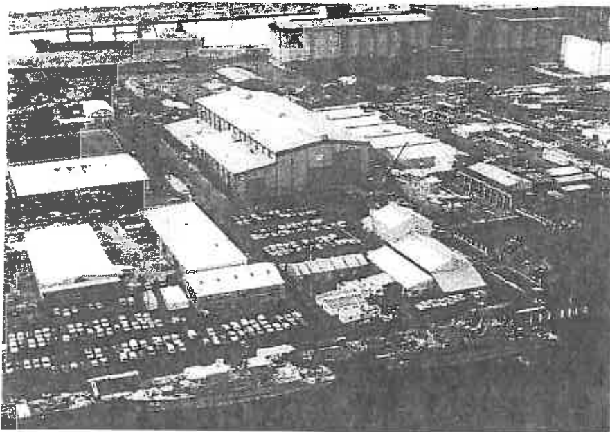
Figure A3.1: The Minehunter Construction site at Carrington, Newcastle, New South Wales
